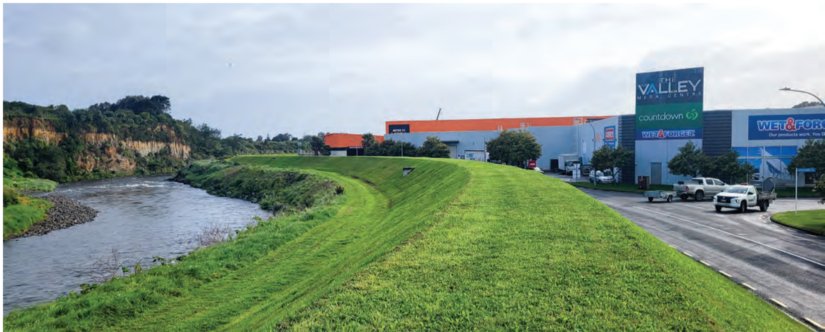
Upgrading to the lower Waiwhakaiho River Flood Control Scheme.
